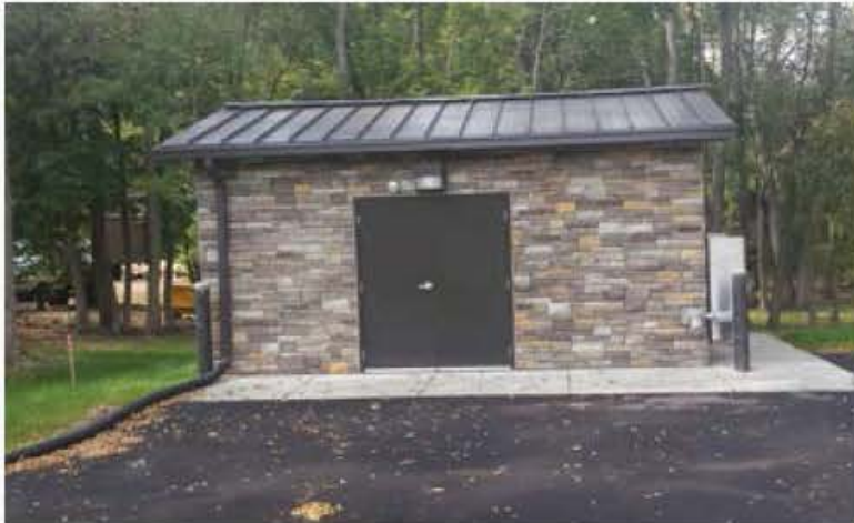
Sample Packaged Booster Pump House
